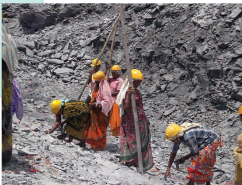
Fig 6.11: Women drilling holes for blasting
