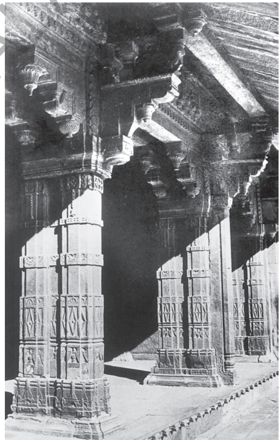
Fig: 22.15 Decorated pillars and struts holding the extension of the roof in Jodh Bai palace in Fatehpur Sikri. They follow the architectural traditions of the Gujarat region.
