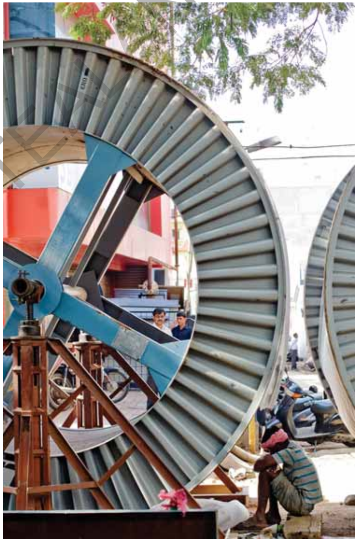
Fig 19.4 Workers laying cables
